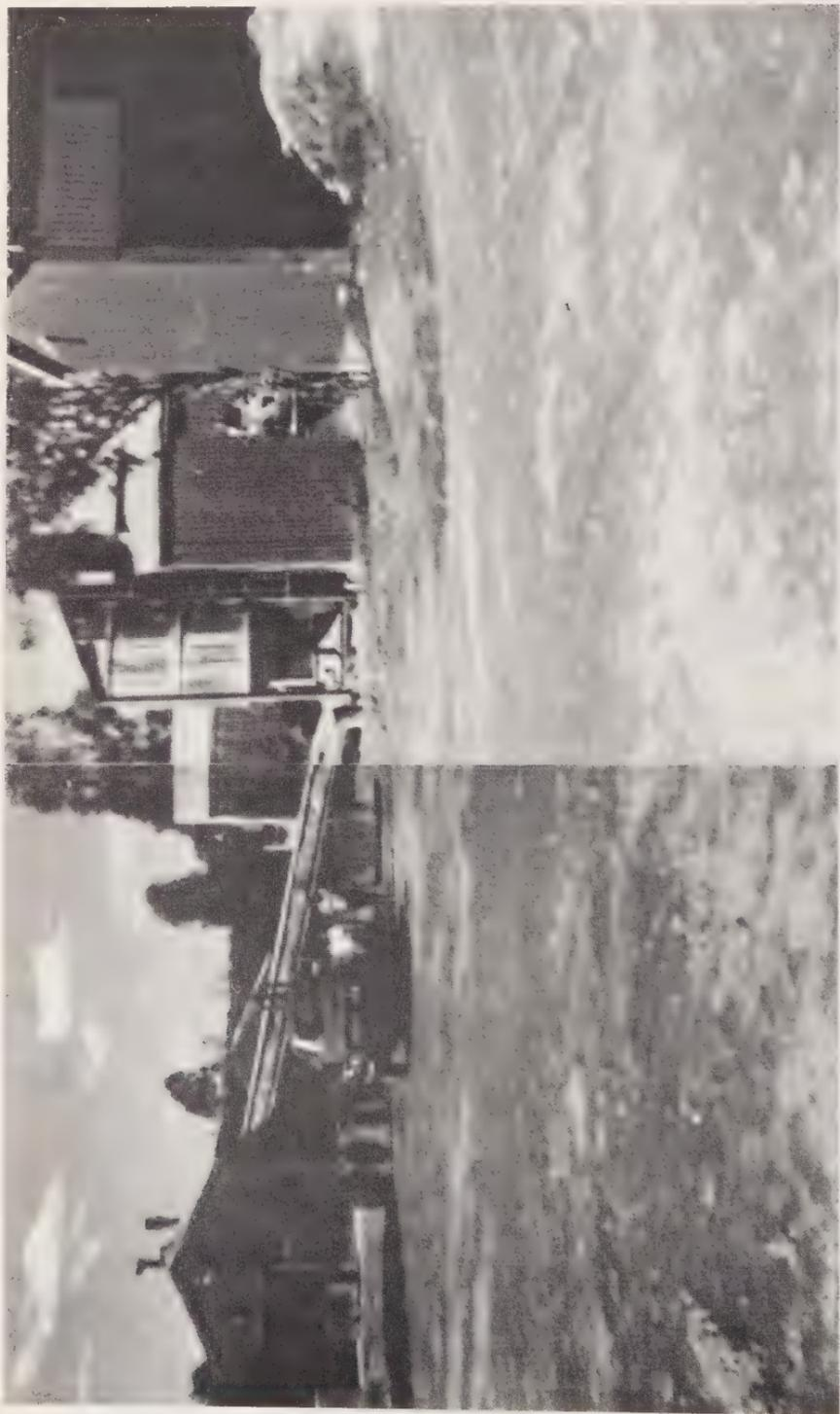
9. The Baryulgil mine in the late 1960s. In the foreground is evidence of the asbestos tailings which were used regularly to dress the roadways in and out of the mill area.
