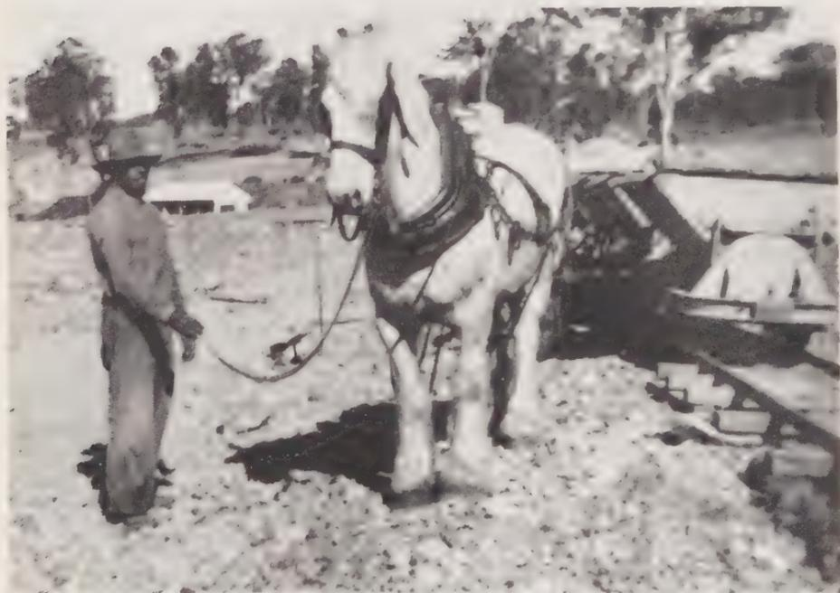
3. During the first years of the mine's operation during World War II, the host rock and tailings were carted by horse-drawn skip from the mine site. This method was used until the end of the 1940s when trucks were introduced.
