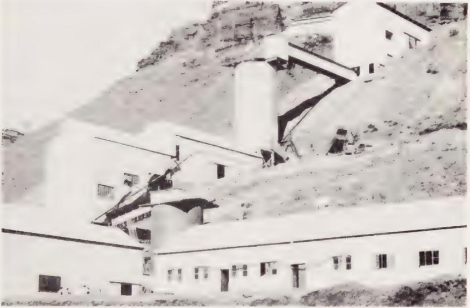
1. The Wittenoom mine was built on three levels down the side of a steep gorge. The crude ore was fed into the mill at the top with the processing taking place at various stages until the fibre had been extracted at the lowest level. At its peak, the mine and mill employed more than 400 men, most of whom were recruited in southern Europe to work for Australian Blue Asbestos.
