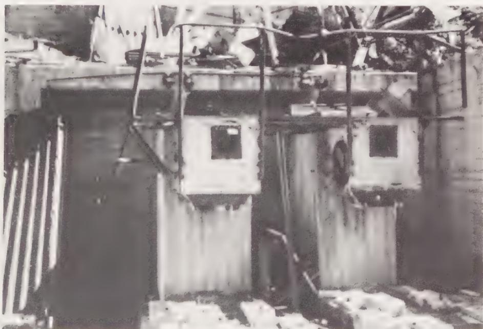
5. The bagging section at the mine, which had been partly demolished when this photograph was taken. This was one of the dustiest sections in the plant, and readings taken by James Hardie officials invariably recorded excessive levels of dust.
