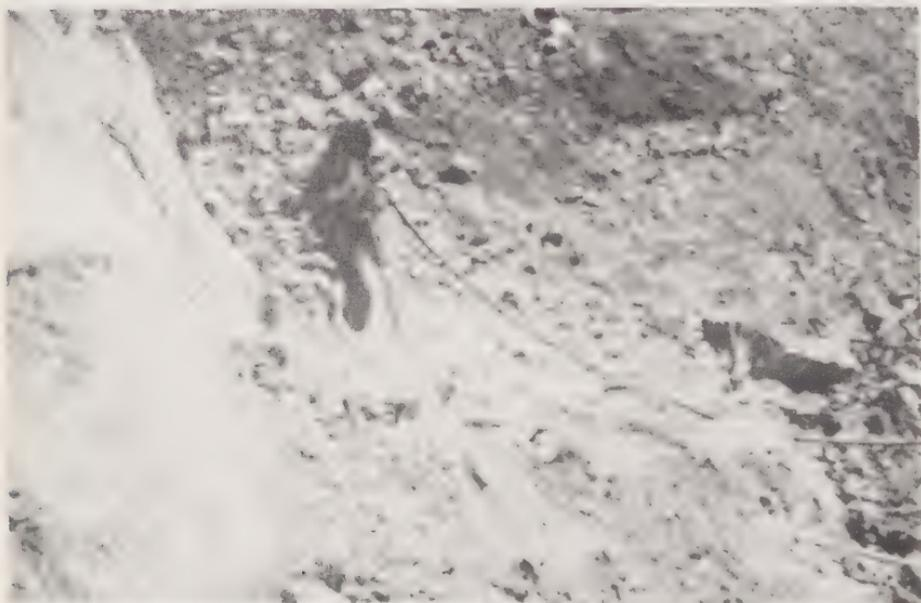
7. The asbestos ore at Baryulgil was mined in an open quarry with drills and the use of high explosives which were used to separate the ore from the quarry face. (Photograph by Mr and Mrs Ken Gordon, Baryulgil)
