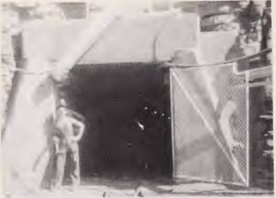
7. The entrance to the Wittenoom mine, c. 1958. The pipe leading into the shaft at the top right conveyed compressed air which was used for drilling.
